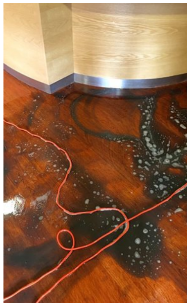
Hard flooring may appear clean to the eye but isn't always clean. The owner of this floor thought the black spots were part of the design – it was in fact dirt.
